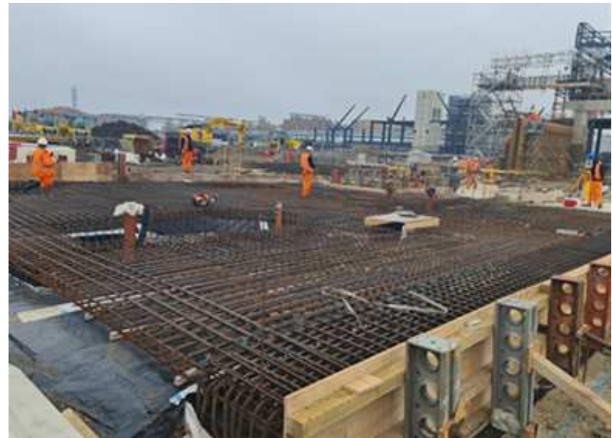
Preparation for concrete pour to the final section of SEEB floor slab
