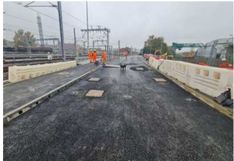
Completed tarmacadam surfacing to the TOC access road and walkways
