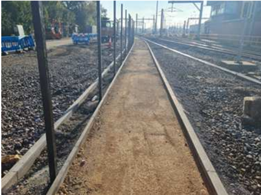
Preparation of the new access road and Drivers Walkway for Tarmac Surfacing
